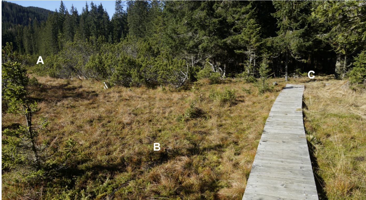
Oblong wooden platform is enough to redirect visitors from former path across the bog (A) to dry bypass (C) through the forest. Fences (rests are slightly notable at B) are not needed any more
